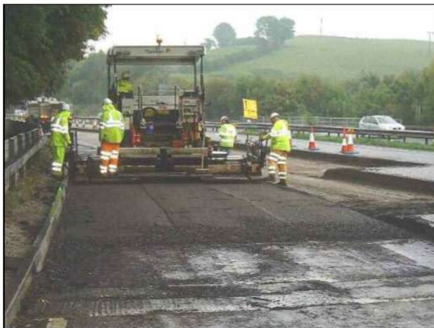
A38 Paving with foamed bitumen base adapted from A38: Ex-situ recycling of a trunk road in South Devon
