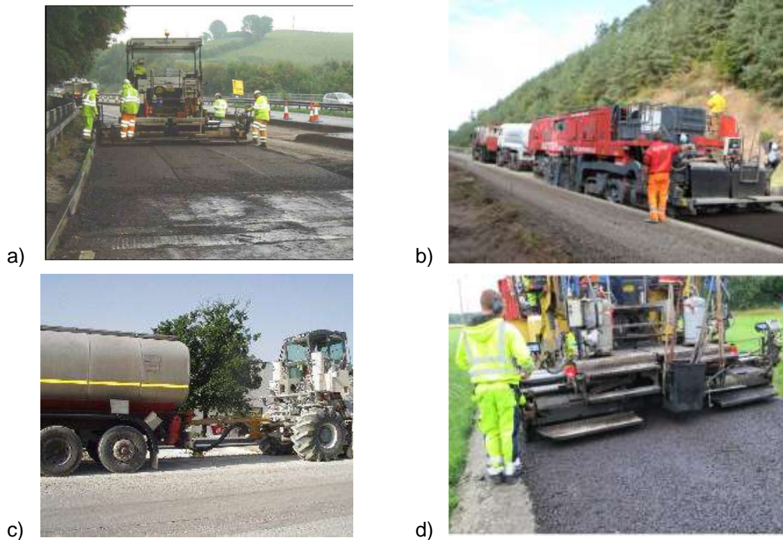
Figure 1. Application of CR techniques: a) CCPR on road A38 in the UK, b) CIR on road B52 in Germany, c) FDR on road SP 18 in Italy and d) CCPR on road Lexby in Sweden.
