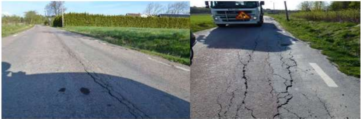
Surface distress before any measures were made.
