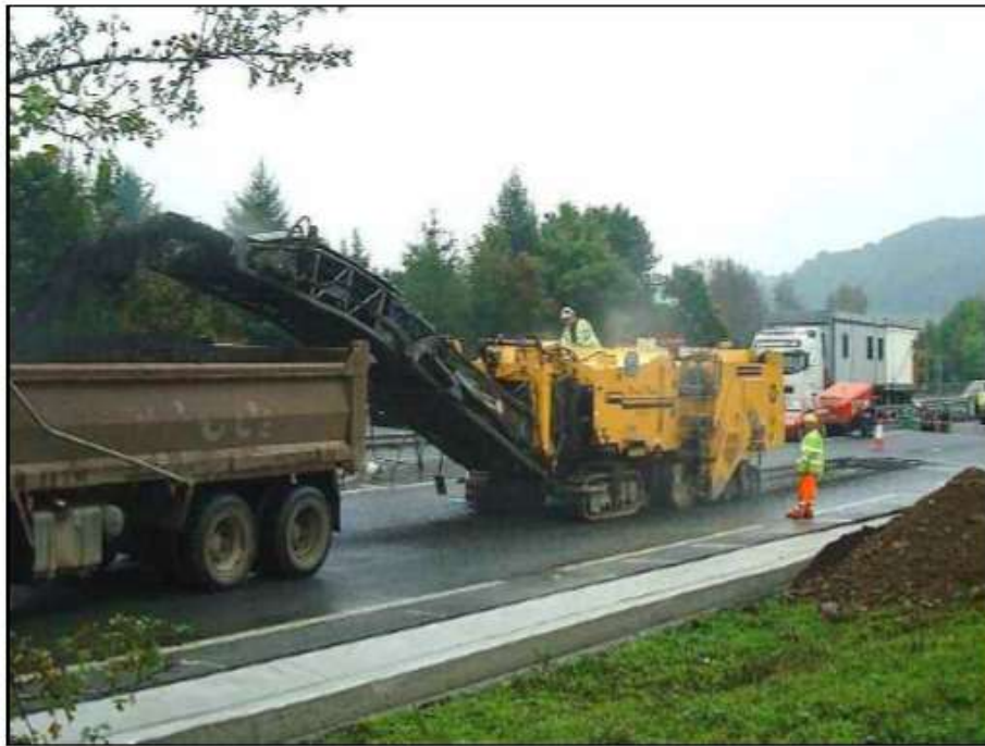
A38 Planning existing pavement base adapted from A38: Ex-situ recycling of a trunk road in South Devon
