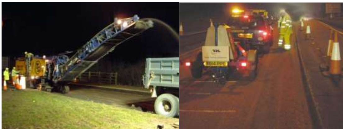
Planning off asphalt (left) and FWD testing (right)
