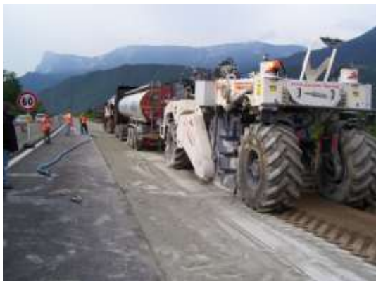
Stabilization with bitumen emulsion
